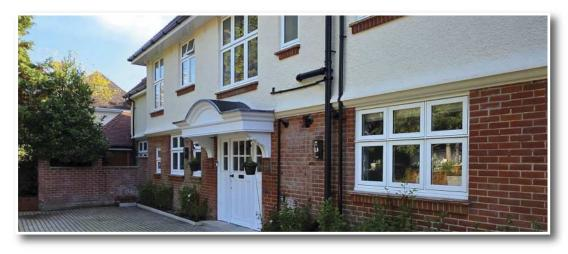
soft, heritage look that complements the property's grandeur inside and out. The installation comprised 54 windows and four French doors, all manufactured using Timberweld and mechanical jointing for authentically butted joints and timber-like detailing. The flush sash exterior and elegant glass sightlines further reinforce the handcrafted aesthetic.
