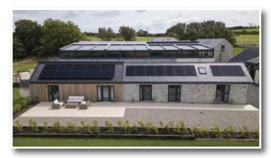
Originally specified in aluminium, the development team transitioned to The Residence Collection after reassessing the design, performance and sustainability goals of the project. The R7 and R2 systems deliver the same clean, flush aesthetic associated with aluminium, while providing significantly improved thermal performance. With u-values as low as 1.2 W/m2K using double glazing,
